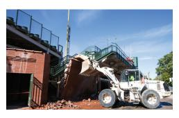
Brandenburg carefully protected the infamous outfield ivy brick wall while removing the concrete stadium seating that was attached to the wall. The crew used equipment that ranged from a large excavator down to handheld demolition equipment including chipping hammers and concrete saws. Bracing was installed
